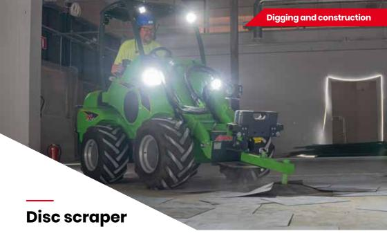
Disc scraper is an excellent and cost efficient tool for removing of carpet and floor tiles in demolition and refurbishing jobs. The durable disc takes off old carpet and tiles quickly and effienctly.
